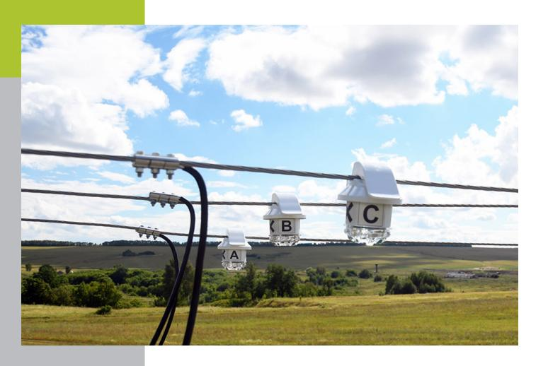
Fault management solution for MV overhead lines Lodestar allows effective localization of fault areas via conductor-mounted indicators of Lodestar CL series, pole-mounted communication equipment Lightbox and software solutions mobile app for on-site configuration & maintenance Lodestar and KOMORSAN Fault Management Software. The system detects all types of faults, collects basic telemetry parameters and transfers the data to KOMORSAN.
